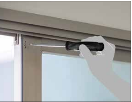
Easily adjustable outer-panel lock
